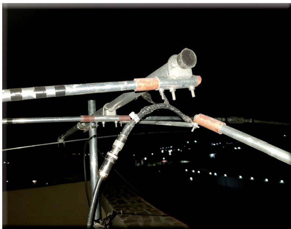
Mosley beam failed!
