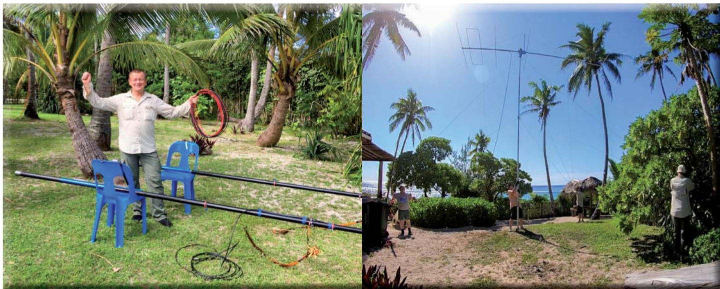
VK5XDX erecting the 40 m 4-square
