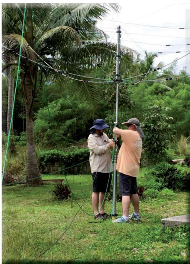
VK5XDX erecting the 40 m 4-square
