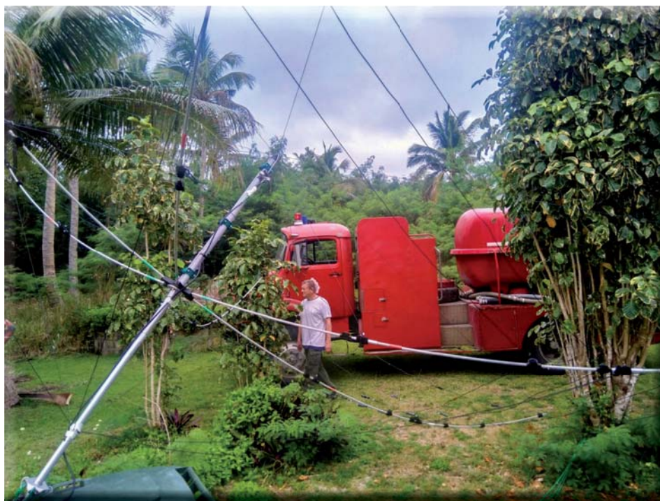
Antennas down and the Fire Brigade in Attendance
