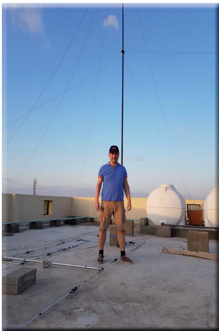
Spiderpole - rooftop extension - sloping wires to ground level
