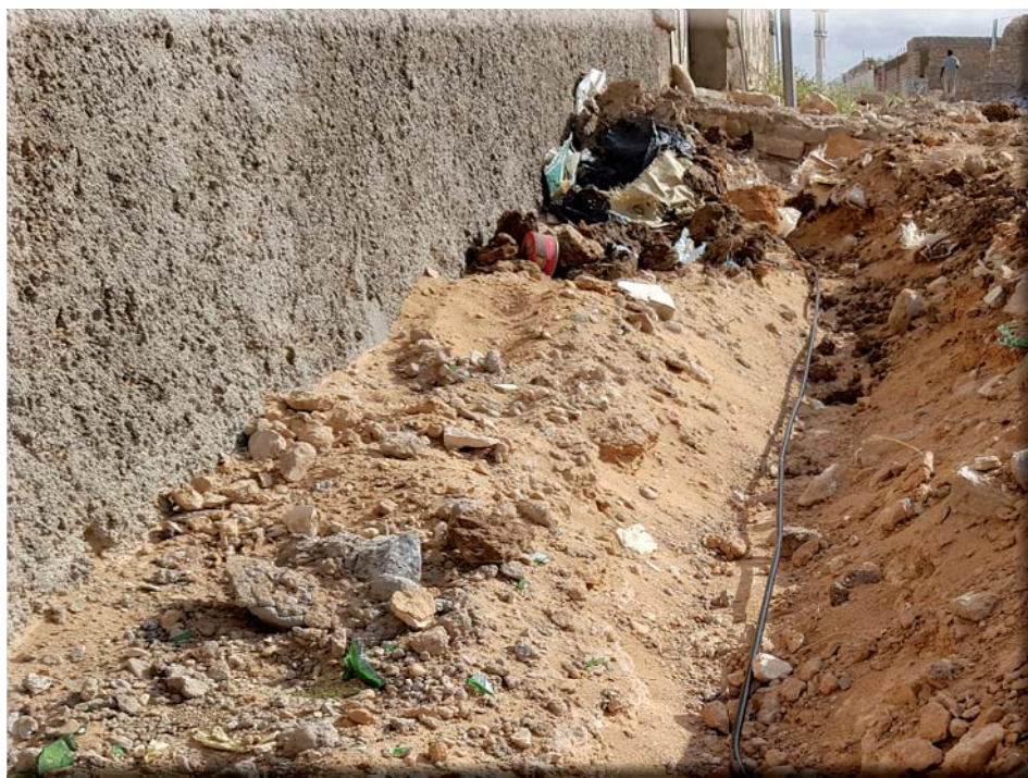
Trench dug by local craftsmen 4" deep!
