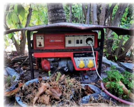
The Honda-3 generator
