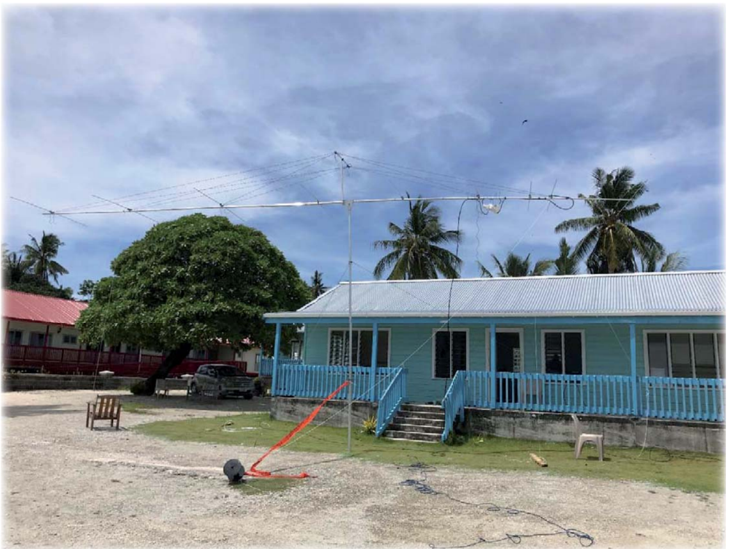
On arrival, the main team just installed a delta loop for 160 m hanging from a cellphone tower on the island and a 9 element beam for 6 m.
