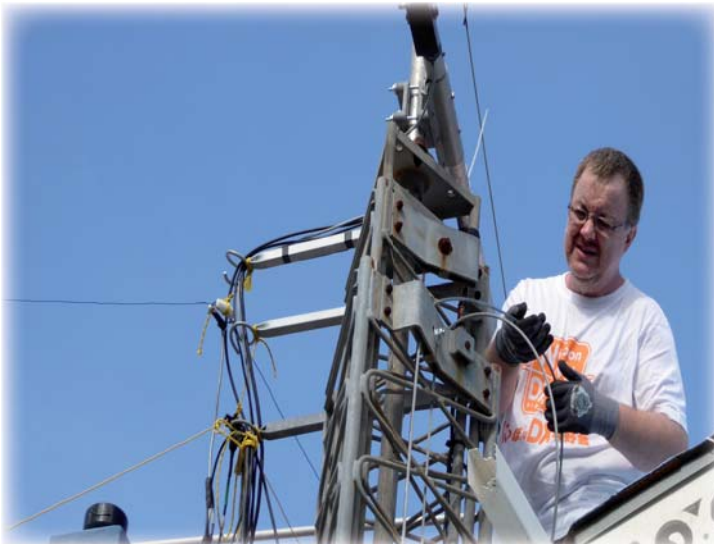
The tower is repaired! DL7UFR changing the steel guy wires. This should keep at least for another 10 years!
