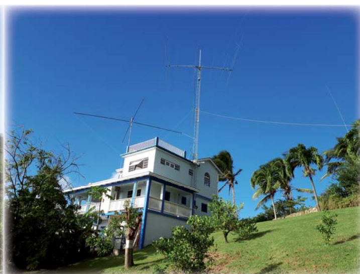
VP2MDL QTH: TH6 yagi mounted on top of the antenna mast and a spiderbeam attached to the balcony.
