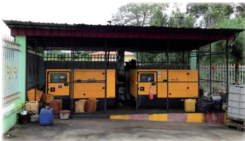
Two 36 Kw generators
