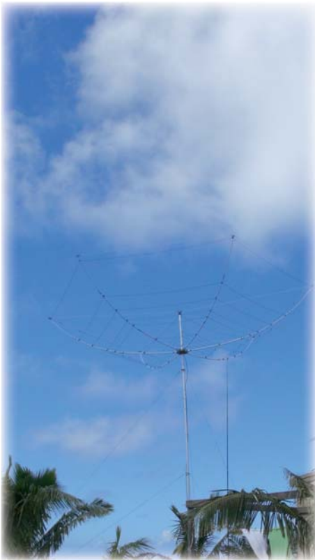
Hexbeam and 30 m vertical
