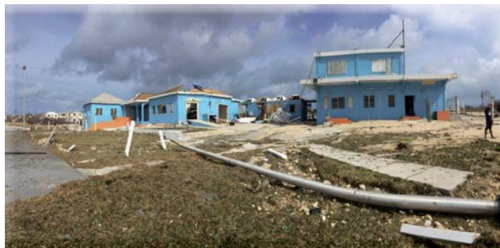
Blowing Point Ferry Terminal.
