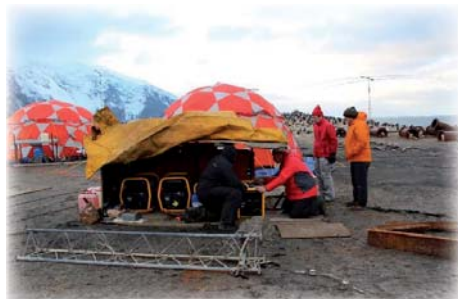
The Team troubleshoots a generator issue amid the ruins of the Argentine base.
